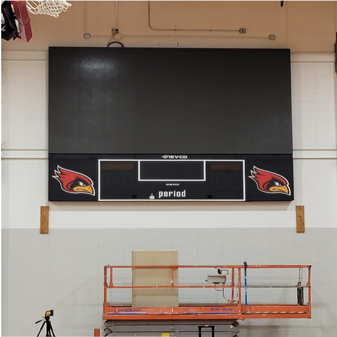
Raytown South High School Score Board Installation
