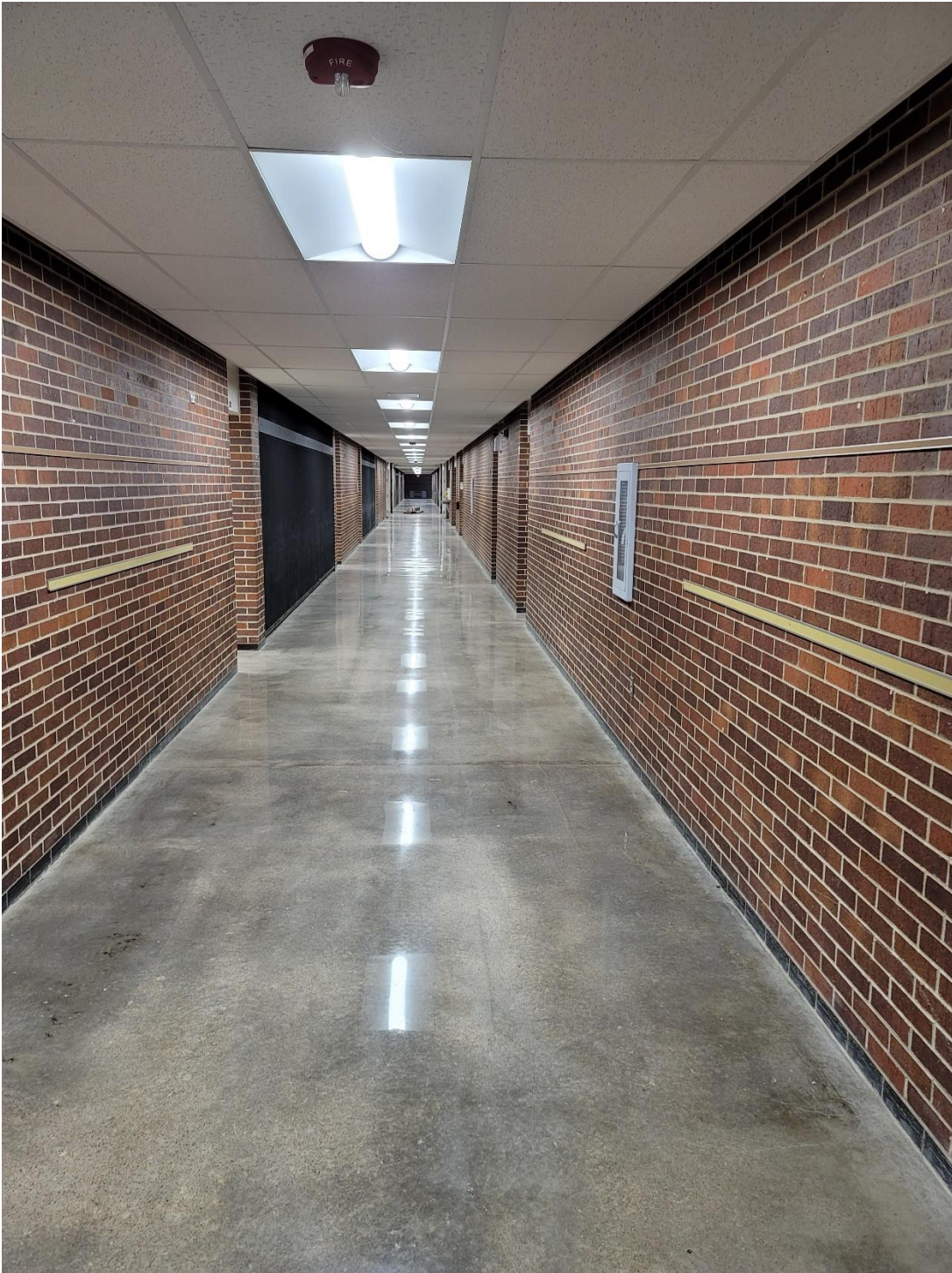
Fleetridge Elementary School Polished Concrete Floors
